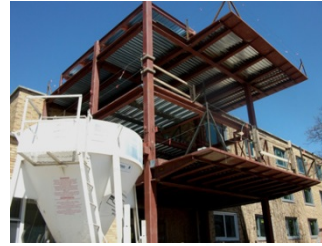
While under Construction
